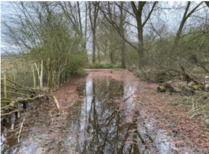
CH1565-CH1645 localised flooding of the Sustrans downstream of the bridge is caused by waters backing up from the choked Redhill Brook alongside, dredging and debris clearance from the Redhill Brook is recommended to relive the flood risk.
