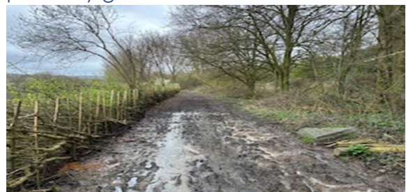
CH1645-CH1953 localised surface flooding (can be addressed with Redhill Brook dredging and clearance), then remove surface debris and mud, place MOT Type 1 raise by 150mm, and top with 8mm to dust pathway gravel.
