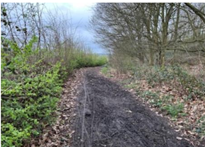
CH1645-CH1953 localised surface flooding (can be addressed with Redhill Brook dredging and clearance), then remove surface debris and mud, place MOT Type 1 raise by 150mm, and top with 8mm to dust pathway gravel.
